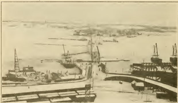
FIG. 1. OLD BRIDGE AND TEMPORARY STRUCTURE.
